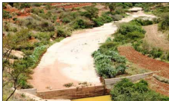
FIGURE 6 Sand dams store up to 30 million liters of water and create the opportunity to invest in ecological agriculture
